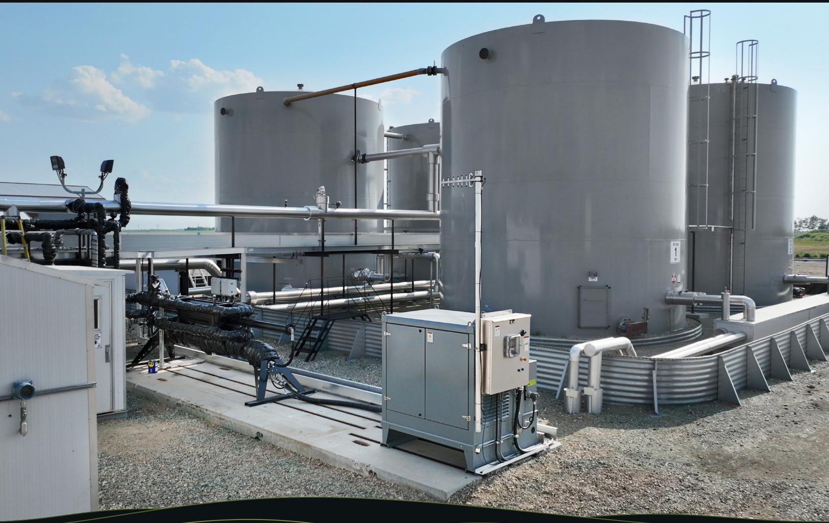
**IJACK VRU** AUTOMATED VAPOR RECOVERY UNIT IS DESIGNED TO REMOVE VAPOR GAS FROM INSIDE TANKS AND VESSELS, ENSURING THAT INTERNAL PRESSURE IS MAINTAINED AT A PRE-SET TARGET LEVEL. BY ENTERING THE MINIMUM AND MAXIMUM TANK/VESSEL PRESSURES, THE VRU AUTOMATICALLY ADJUSTS ITS SPEEDS TO ACHIEVE AND MAINTAIN THE REQUIRED PRESSURE.
